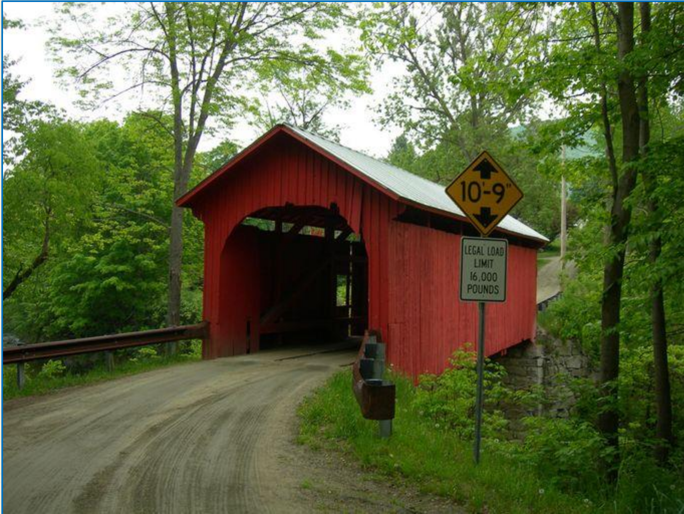
Crossing the Dog River in Northfield, Vt., is the Slaughter House Covered Bridge. It was constructed in 1872 and uses the Queen post truss design
