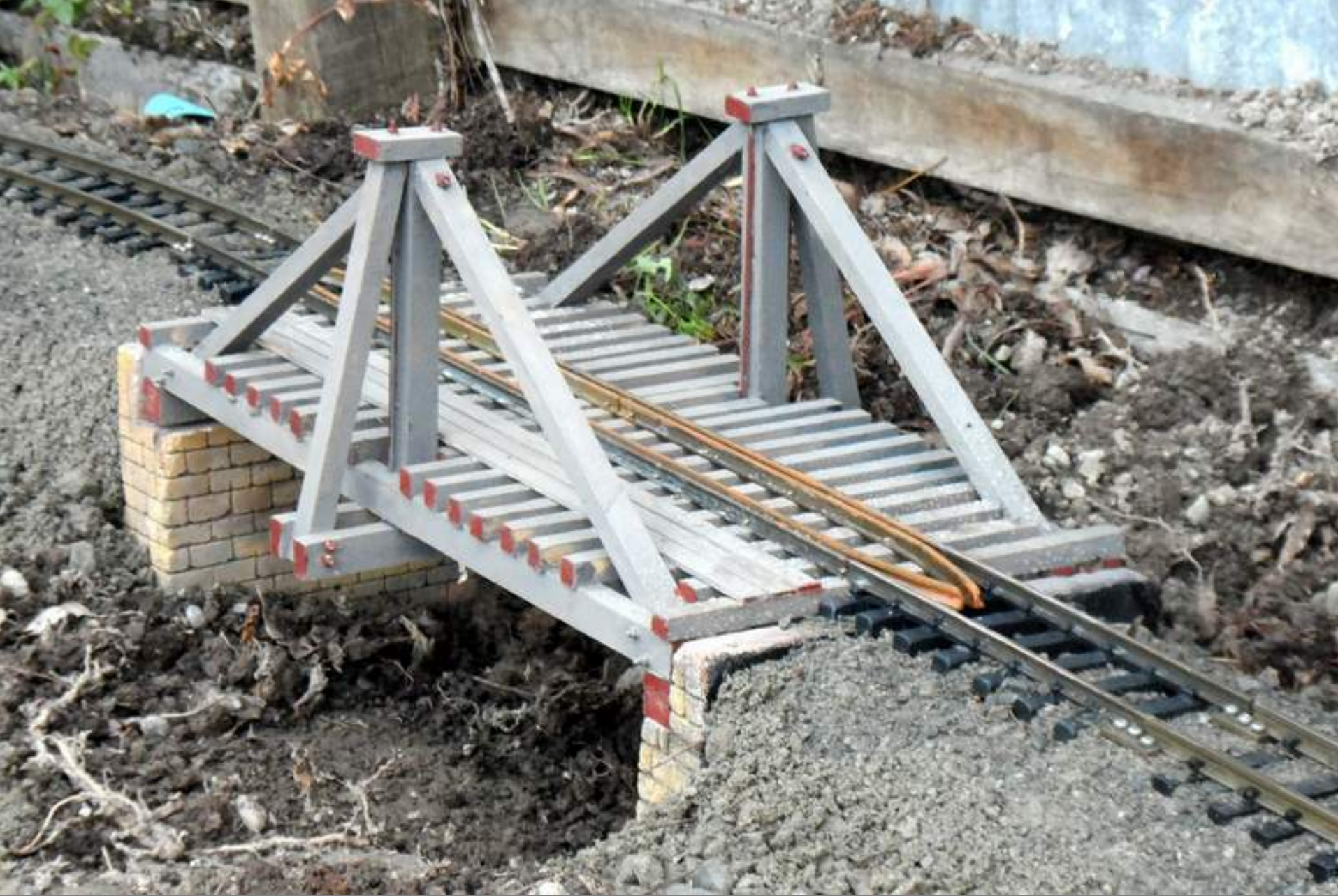
The King Truss Bridge is completed and installed. The Abutments are made of Hebel Concrete scribed to represent block construction and coloured to match natural rocks elsewhere on the railway.
